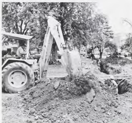
Workmen prepare trenches for new water lines.
