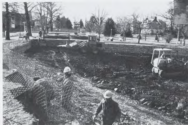
Since the 1950s, the stone lake wall has looked much like this 1970s photo. At left, workers build wire cages, which were later filled with stone to create the lake's new gabion wall.
