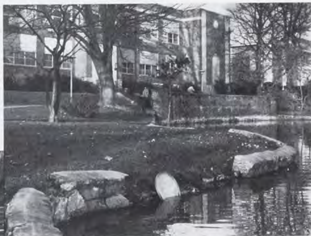
Despite continual repairing and rebuilding, the lake wall often fell victim to the freezing and thawing of Lancaster's winters.
