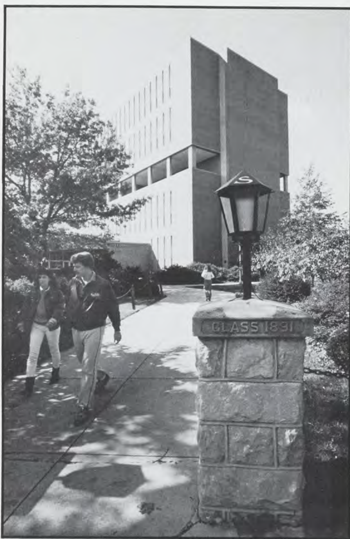
The high-rise Ganser Library dominates the center of the Millersville campus.
