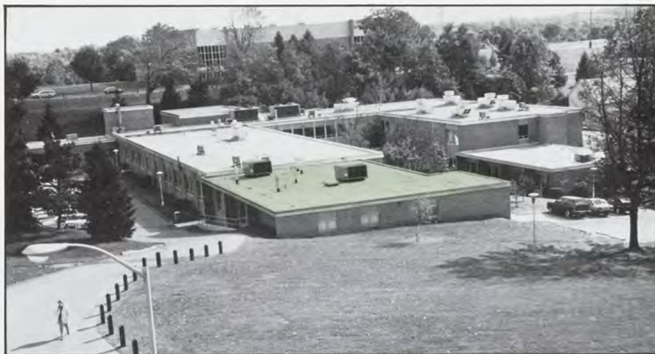
The green shaded area is the addition, now extending the north wing of the second floor of Roddy Science Center westward, toward Breidenstine Hall. The new facility contains a laboratory, classroom and faculty offices.
