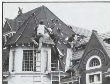
Replacing a leaking asphalt roof with slate is a lofty business.
