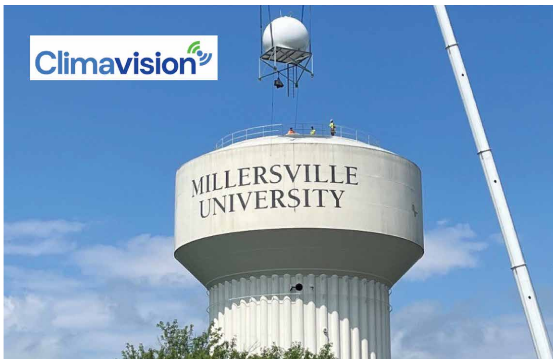
Installation of the Climavision radar on Millersville University's water tower.
