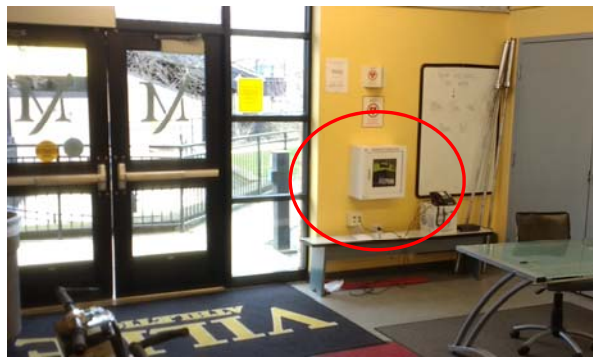
Carpenter-Trout Strength Training Facility. Inside front doors to left
