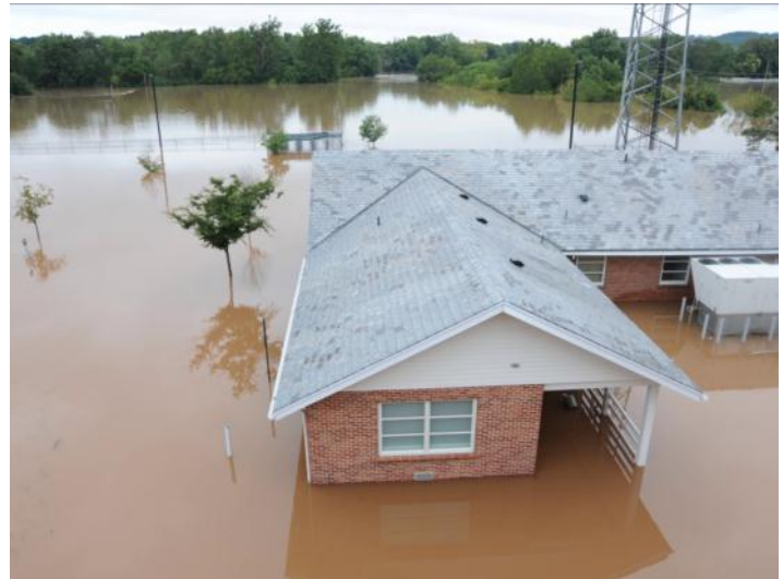
Derry Township Police Department Building with the Swatara Creek at approximately 20 feet. The river crested at 26.8 feet, more than 10 feet above the previous record.
