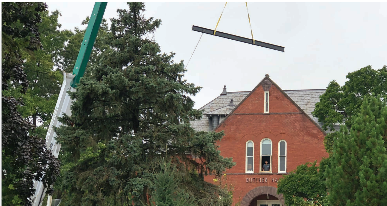
Steel beams being placed in Dutcher Hall by crane.
